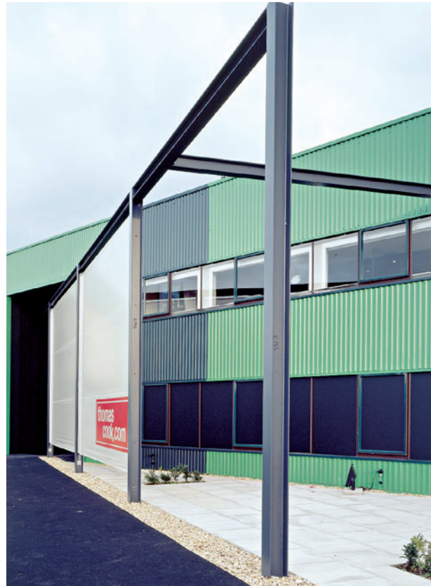
thomascook.com, office fit-out, external view (above)
